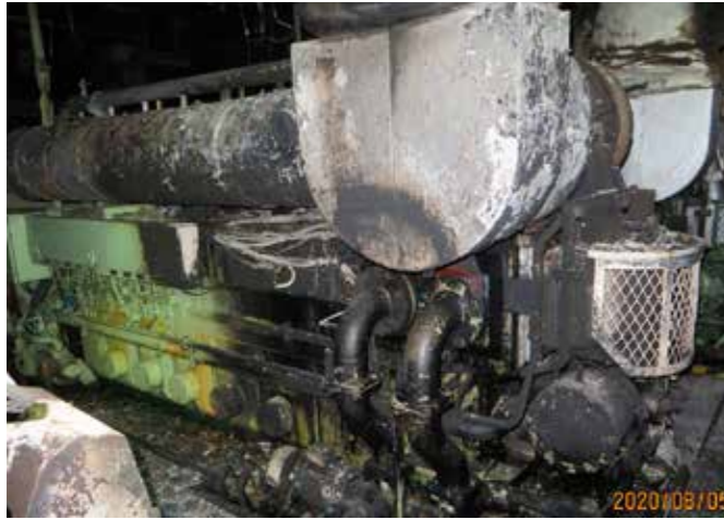
Post-fire AE1 fuel filters
